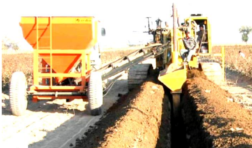
4-rasm. Drenaj quruvchi mashinaing ish jarayoni
